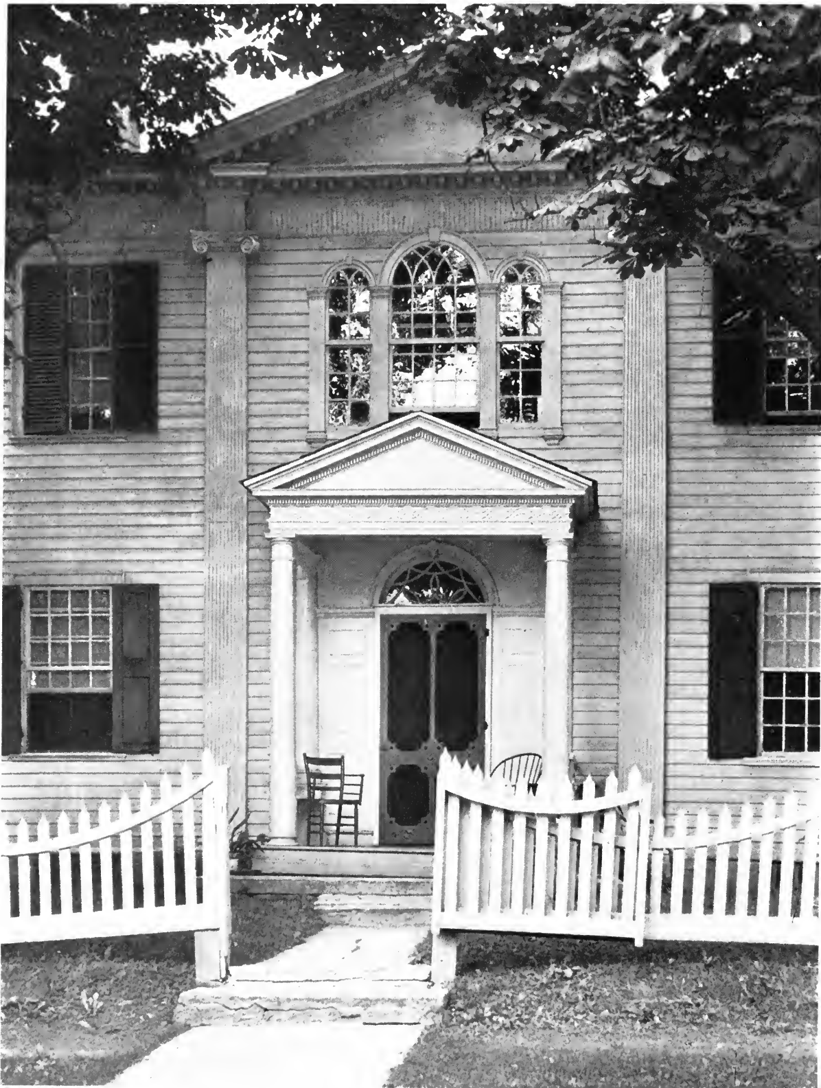
THE GENERAL DAVID ROBINSON HOUSE, OLD BENNINGTON, VERMONT. A unique adaptation of the Palladian window used frequently in the vicinity of Bennington.
