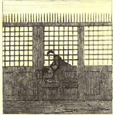
Door leading out of the Chapel .
