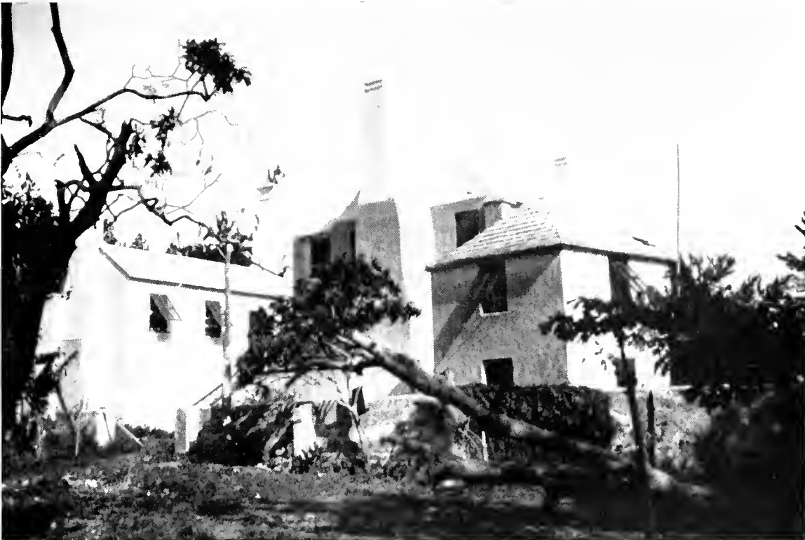
PLATE 51. House in Paget. Side View.
