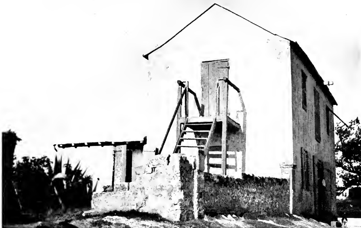
PLATE 52. Shop and Tenement in Warwick.
