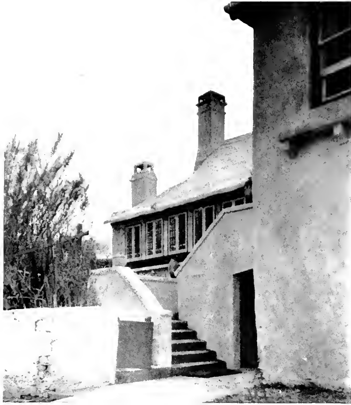
PLATE 55. "The Chimneys," Paget. Road Front.
