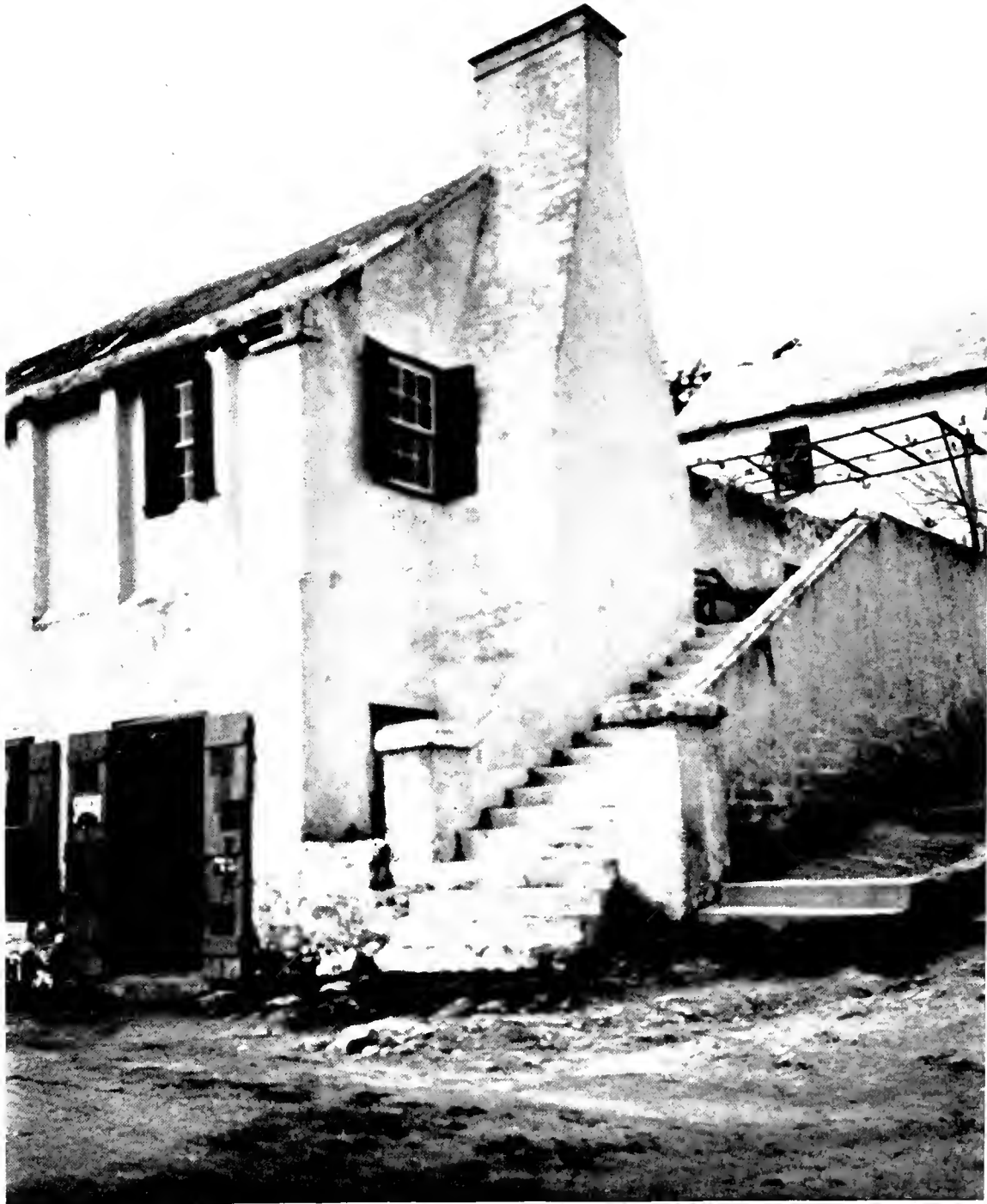
PLATE 137. Shop and Dwelling on Harrington Sound, Smith's Parish.
