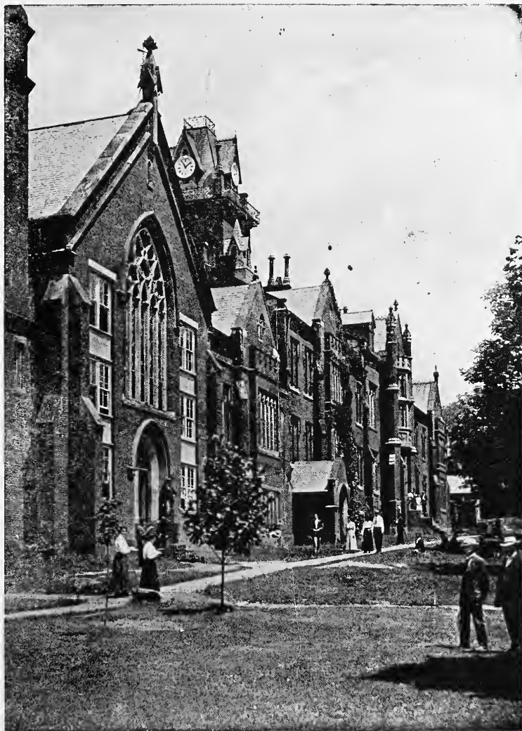
FRONT VIEW OF MAIN BUILDING
