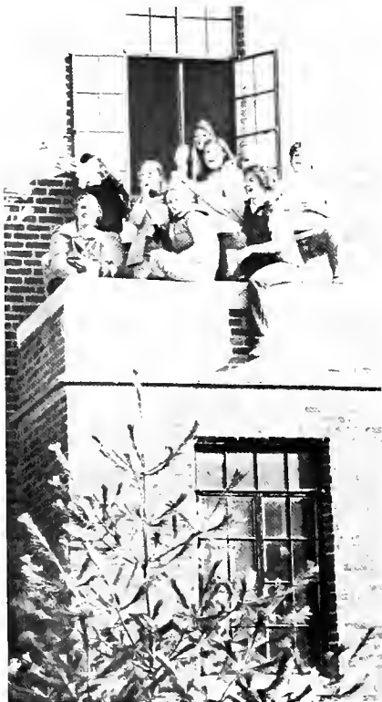
There's safety on the balcony
