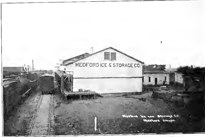
This Medford (Oregon) Ice and Storage Company Warehouse IS INSULATED WITH
