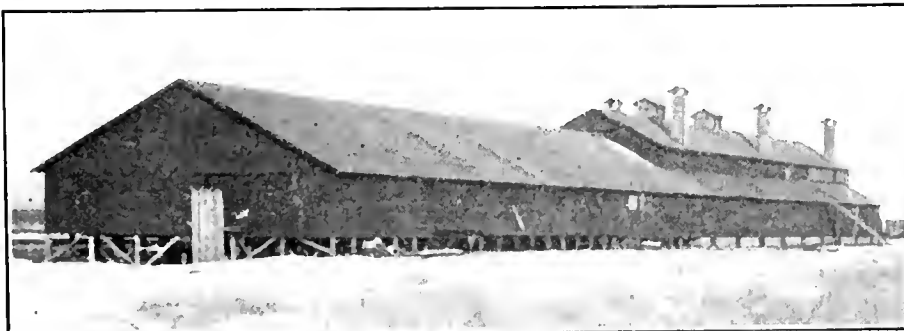
Large type of Northwest apple packing and air cooled storage house. Only the latter, however is frost proof
