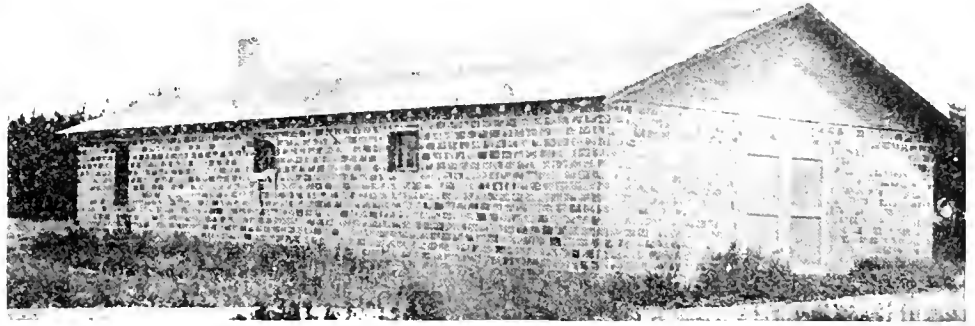
Small type of frost proof Northwest apple packing house. Although constructed of tile, this type of house is both poorly lighted and ventilated.
