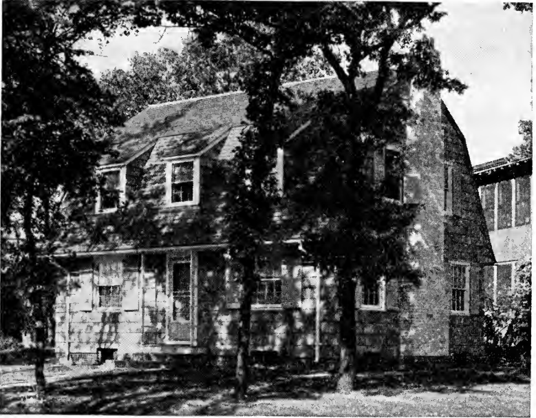
FIG. 16.—Modification of Dutch Colonial house as commonly built to meet modern requirements. Although its double-pitched roof and dormer windows are characteristic of Dutch Colonial style, in the original Dutch Colonials the upper story windows appeared only in the ends of the house. (Copyright—Architects' Small House Service Bureau, Inc., House Plan 6-A-60.)
