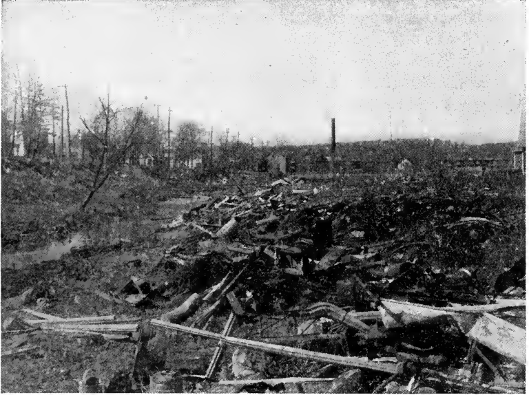
FIG. 72.— Before . Conditions adjoining Main St., White Plains, N.Y., before construction of the Bronx River Parkway. (Courtesy of Planned Progress and Westchester County Park Commission, N.Y.)
