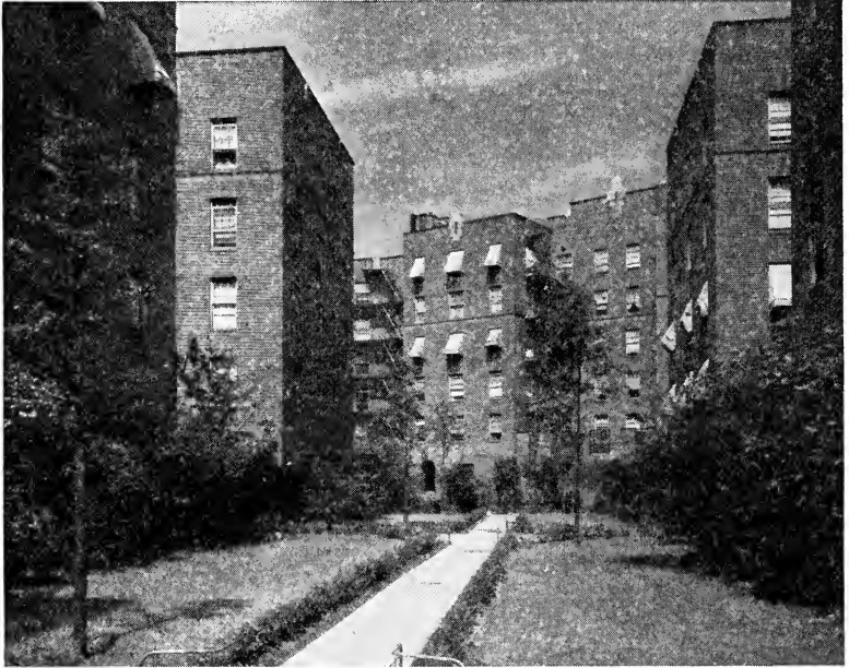
FIG. 77.—Paul Lawrence Dunbar Apartments for Negroes, Harlem District, N.Y.—a John D. Rockefeller, Jr., project.
