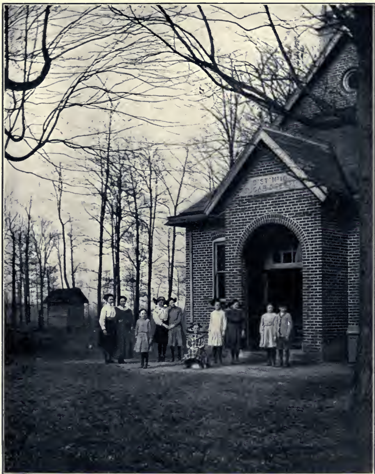
This building was planned for a school of forty or fifty pupils. The attendance has now dwindled to nine. For two years the boy shown in the picture was the only boy in the school. This is a case where a good district building adequately equipped fails to attract pupils when a consolidated school is within reach
