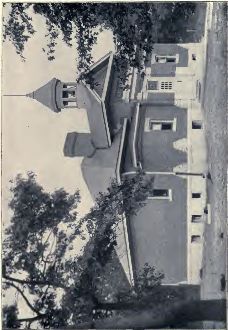
A model district school. Lighted from the north. Basement under entire building. Heated by furnace. Spacious hallways, cloak rooms; toilet inside; plenty of playground. Cost $4,200 Courtesy of H. L. Rogers (Ind.)
