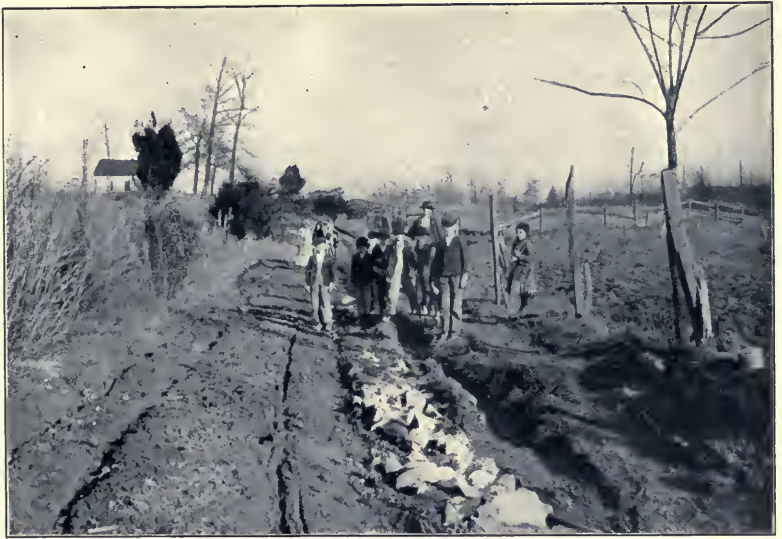
The bad road
