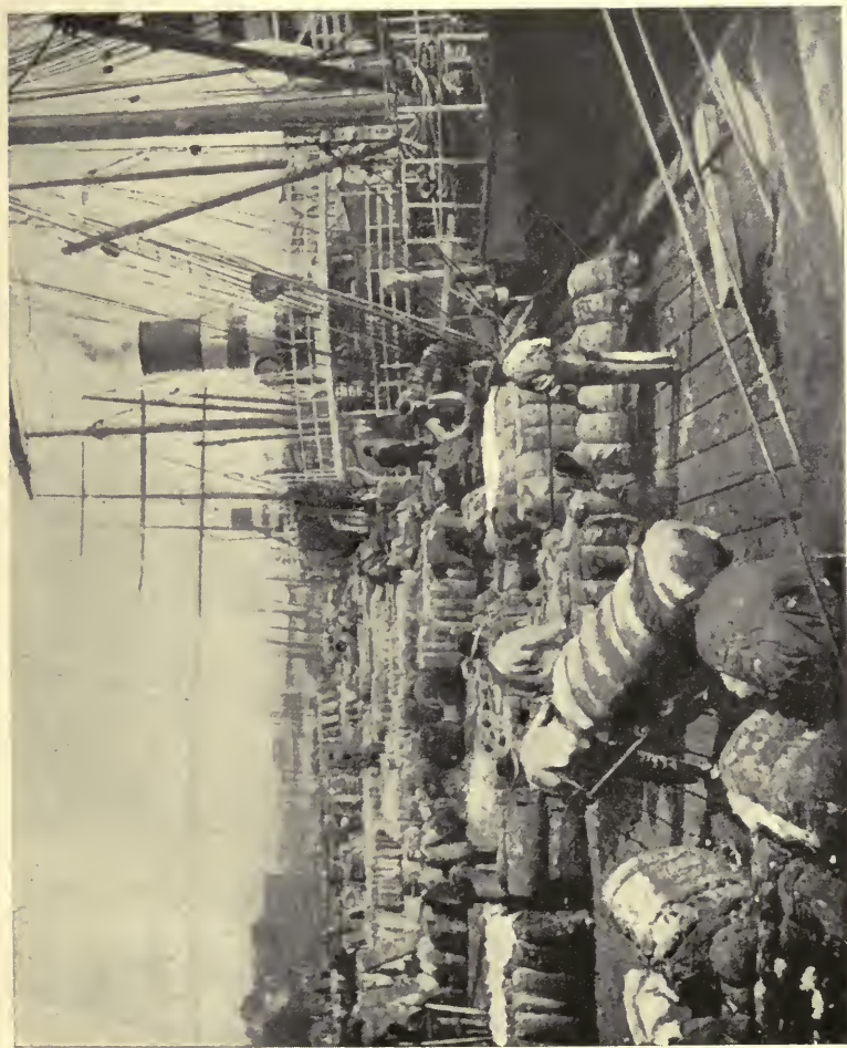
THE LEVEE, NEW ORLEANS
