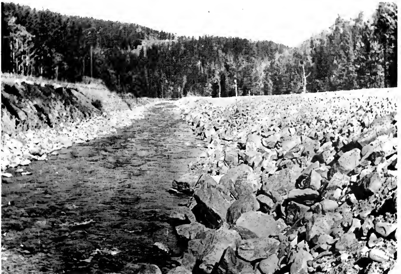
POOR STREAM HABITAT... Straightened to accommodate the highway at right.
