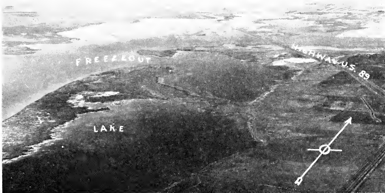
Construction of an outlet canal, representing the initial phase of development of Freezout Lake, was begun during the biennium.
