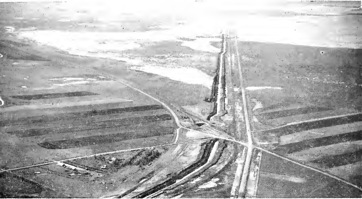
Freezeout Lake showing drainage ditch constructed in this largest waterfowl habitat development project yet undertaken by the Fish and Game Department.
