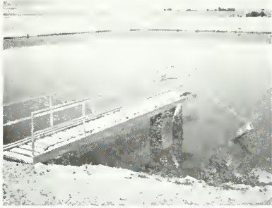
Sewage Lagoon pictured above treats human sewage.
