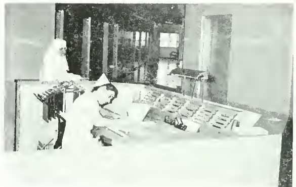
Nurses' station in a newly constructed Montana hospital is pictured above.
