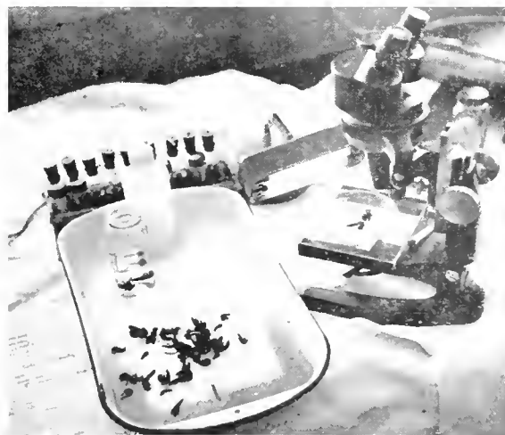
Staff collects river bottom organisms and the organisms found are identified and typed. This determines the degree of river pollution
