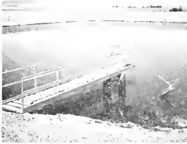
Sewage Lagoon pictured above treats human sewage.
