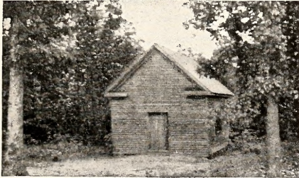
BARTON'S CREEK TOWNSHIP Districts Nos. 2 and 5, Consolidated
