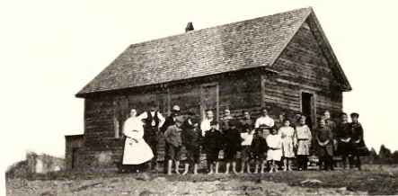
MT. HOPE District No. 6, St. Mary's Township, old building
