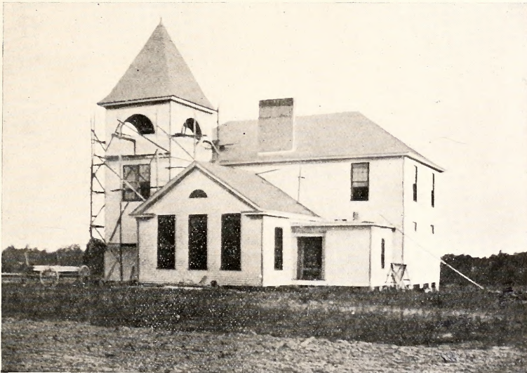
THE NEW BUILDING AT GARNER UNDER CONSTRUCTION
