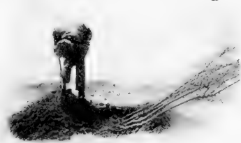
"HEELING IN" OPERATION COMPLETED, EXCEPT SHOVELING SOIL IN PLACE
