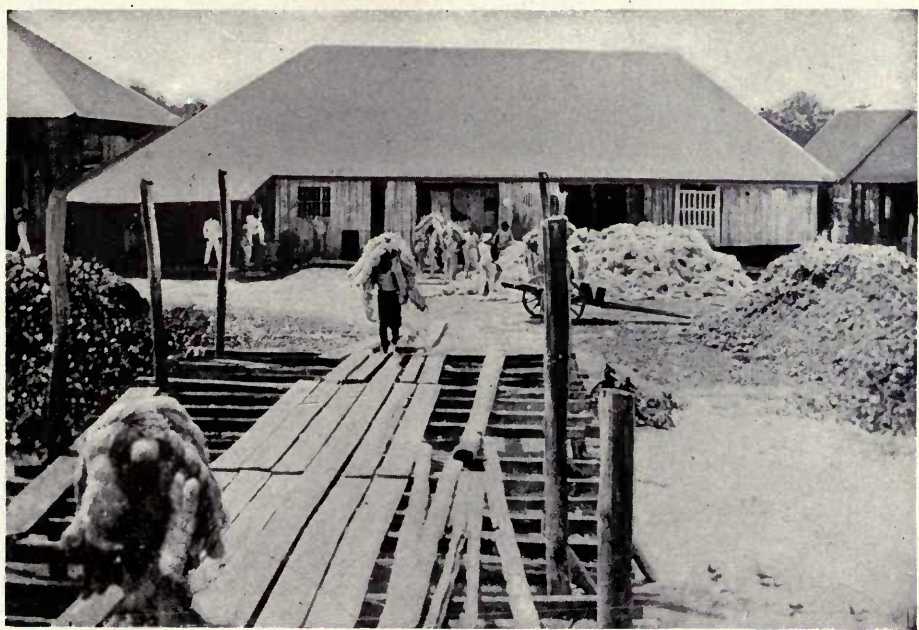
Carrying Fibre to the Wharf
