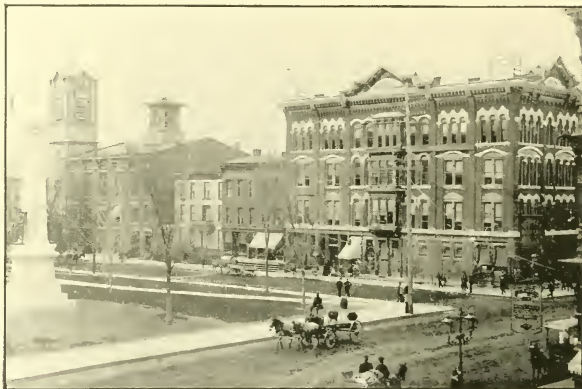
COLLIER STREET LOOKING SOUTH.
