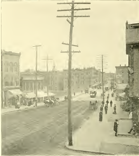
MAIN STREET, AND COURT STREET BRIDGE.
