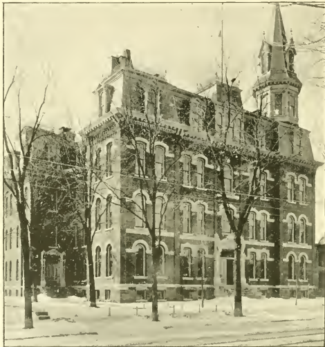
BINGHAMTON CENTRAL HIGH SCHOOL.
