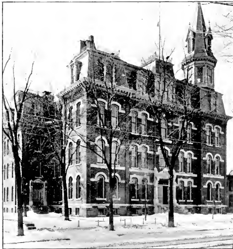
BINGHAMTON CENTRAL HIGH SCHOOL.
