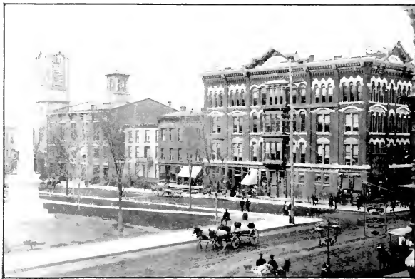
COLLIER STREET LOOKING SOUTH.
