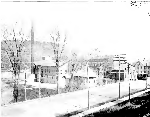
POWER STATION AND CAR HOUSE OF THE BINGHAMTON RAILROAD CO.
