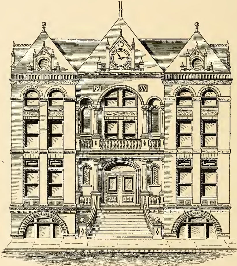
CITY HALL OF DOVER.
