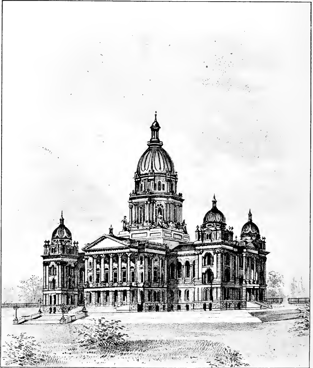
IOWA STATE HOUSE AT DES MOINES.
