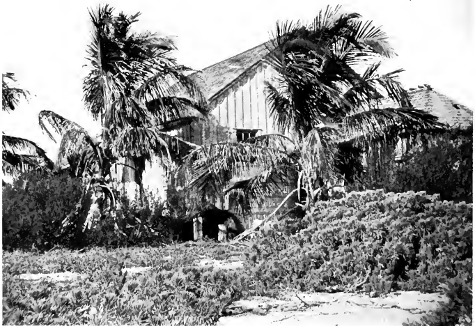
OLD HOSPITAL BUILDING, BIRD KEY, DRY TORTUGAS, FLORIDA Used by wardens as a residence
