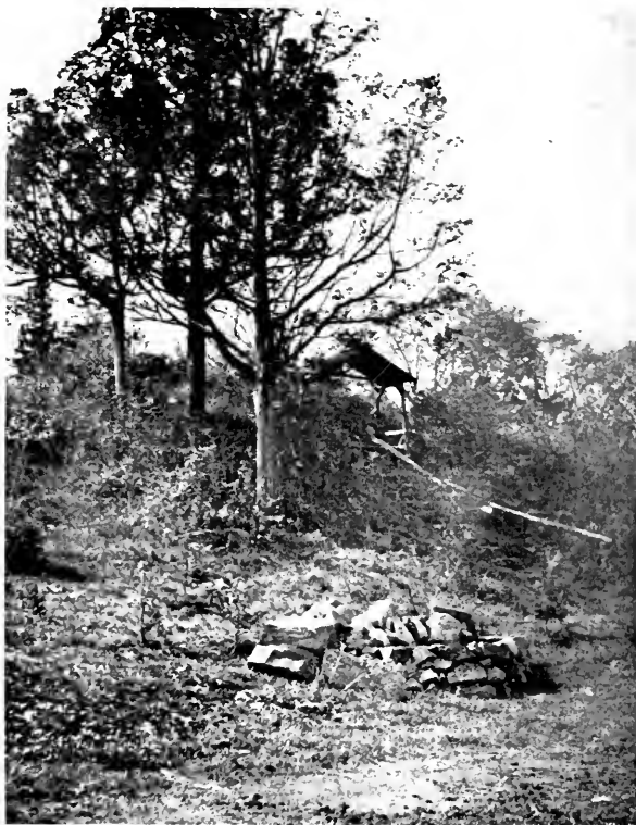
A ROUGH STONE BATHING-Pool AND OBSERVATION SHELTER
