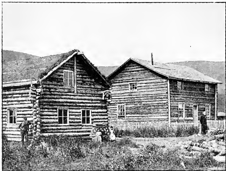
See House and Storeroom of Bishop Bompas.
