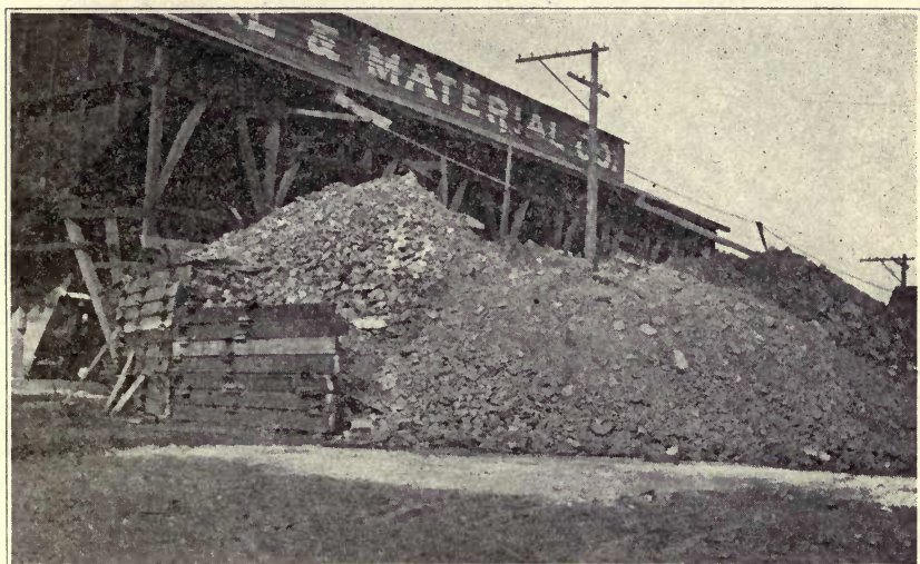
FIG. 25. VIEW OF COAL PILE SHOWING TIMBER RETAINING WALL ANCHORED INTO COAL PILE BY WOODEN SUPPORTS
