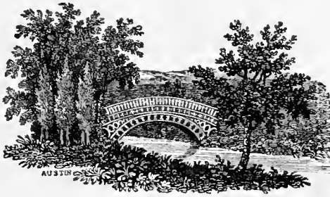
IRON BRIDGE IN LEE VALE.
