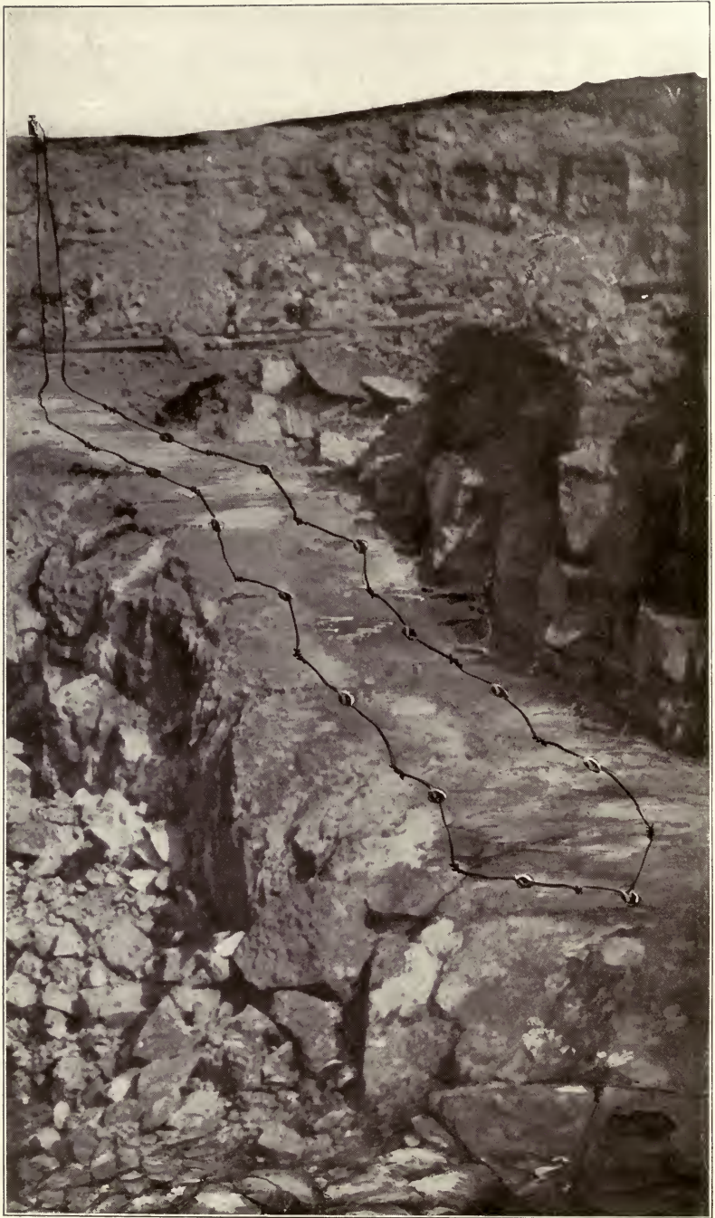
Blasting Circuit Connected in Series
