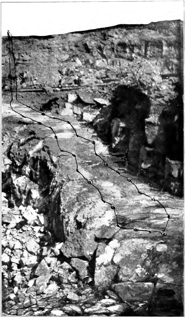
Blasting Circuit Connected in Series
