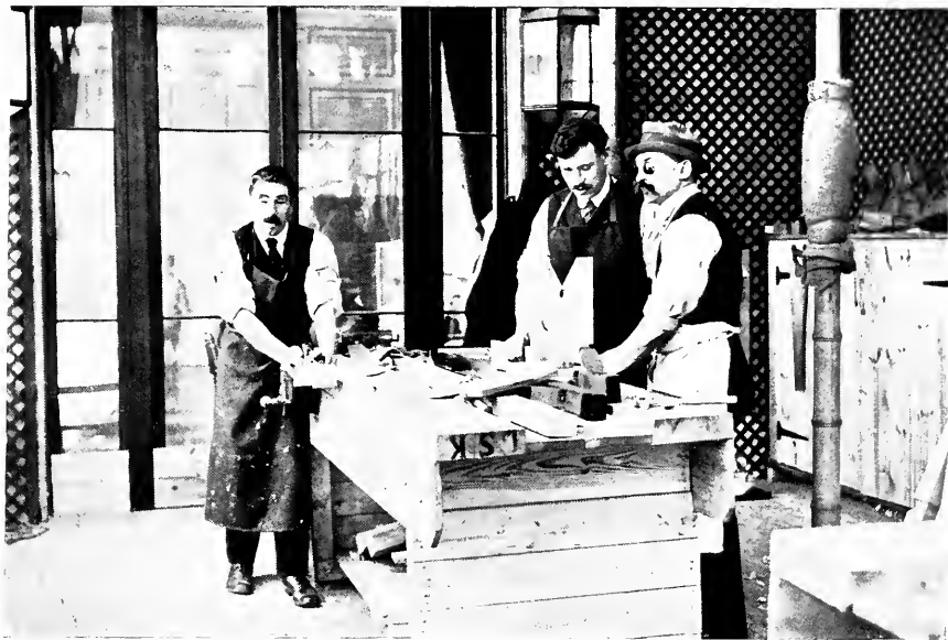
IN THE CARPENTERS' SHOP. (At the Blinded Soldiers' and Sailors' Hostel.)
