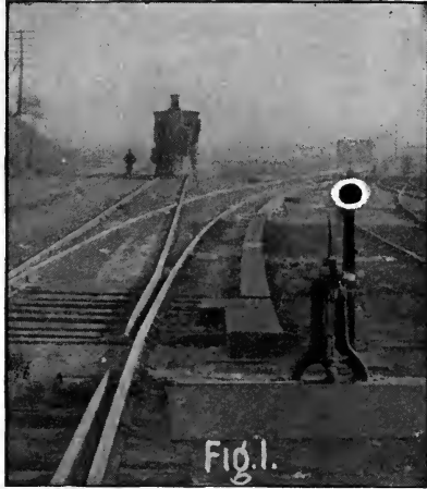
SWITCH TARGET USED TO INDICATE DANGER.
