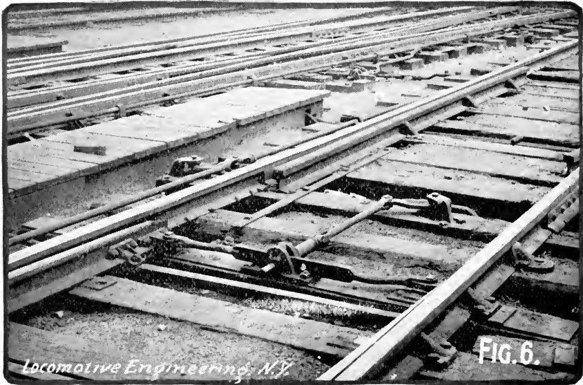
INSIDE-CONNECTED FACING-POINT LOCK.
