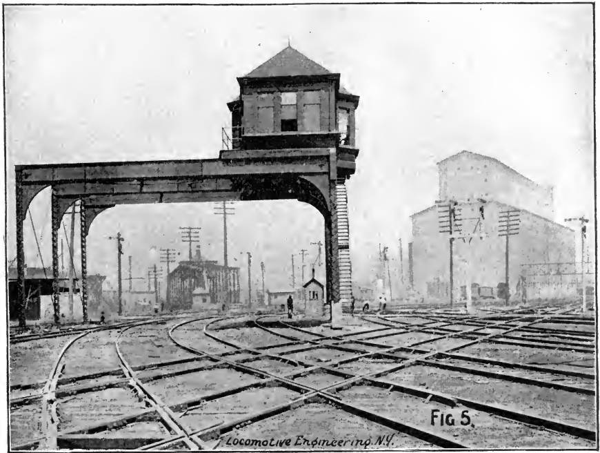
TOWER HOUSE FOR ELECTRO-PNEUMATIC INTERLOCKING MACHINE.
