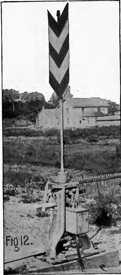
ELLIOTT'S ELECTRICALLY-LOCKED SWITCH STAND.
