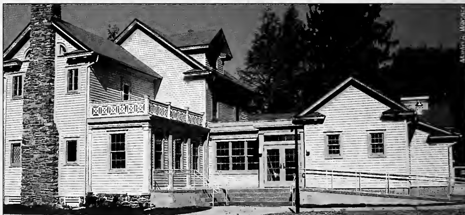
The Fenstemaker Alumni House doubled in size with the completion of a 2,700-square-foot addition. Featuring a great room named in honor of the late Curtis R. English, former university president, the addition was dedicated during Homecoming Weekend. Funded by the Alumni Association and Bloomsburg University Foundation Inc., the $480,000 project includes two accessible restrooms, a kitchen, coatroom and storage area. The Fenstemaker Alumni House, shown from the parking area, has been home to the Alumni Association since 1985.
