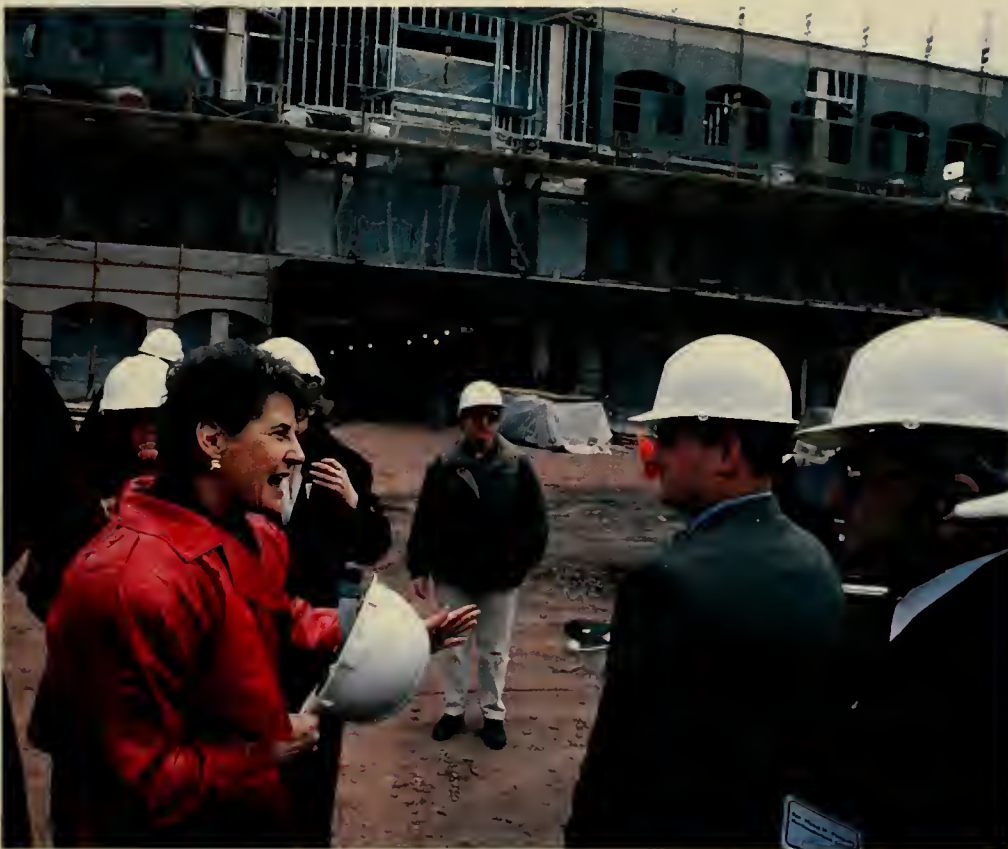
BU's current president, Jessica Kozloff, left, checks progress during construction of the 'new' Andruss Library.
