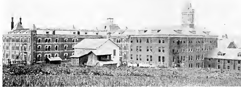
The original barn, related outbuildings and a field of corn and cabbage can be seen in the foreground in this 1893 photograph. In the background is the dormitory complex, later Waller Hall.
