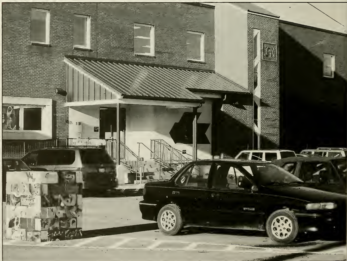
The Studio Center is across South Main Street and offers students a better environment. This building was a necessary addition for the school of Art & Art History. ■ Photo by Rachel O'Donnell
