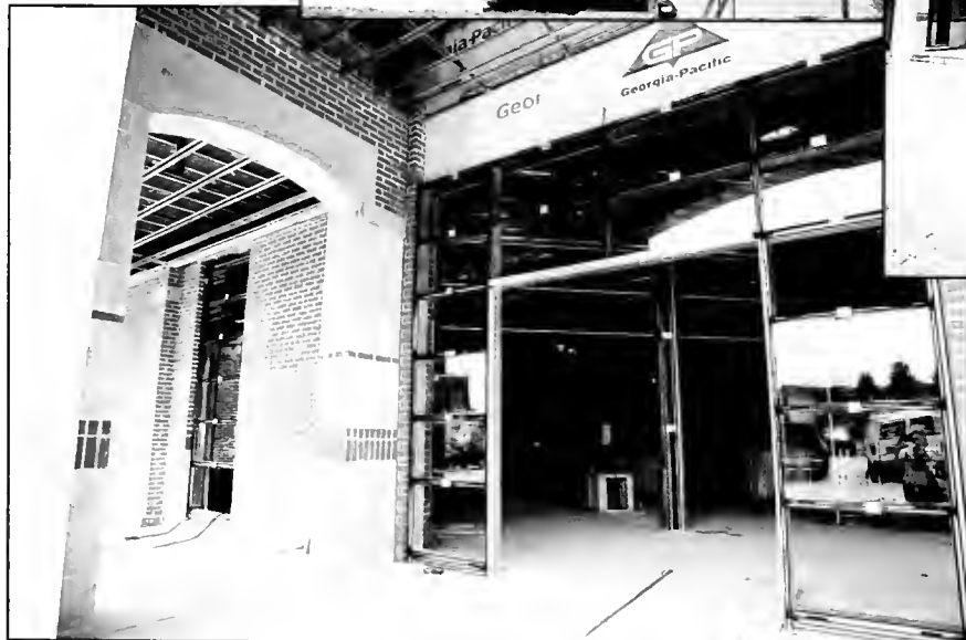
Transforming from a faculty parking lot in front of Godwin, to a brand new bookstore, the construction began in Spring 2002. The two story building was expected to be completed before the end of the fall semester. • Photos by Rachel O'Donnell and Jenny Brockwell
