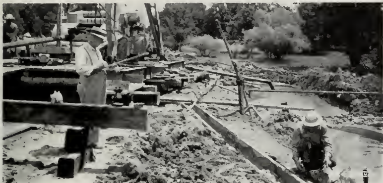
"Catching samples" of drill cuttings at a well for study of possible producing reservoirs.
