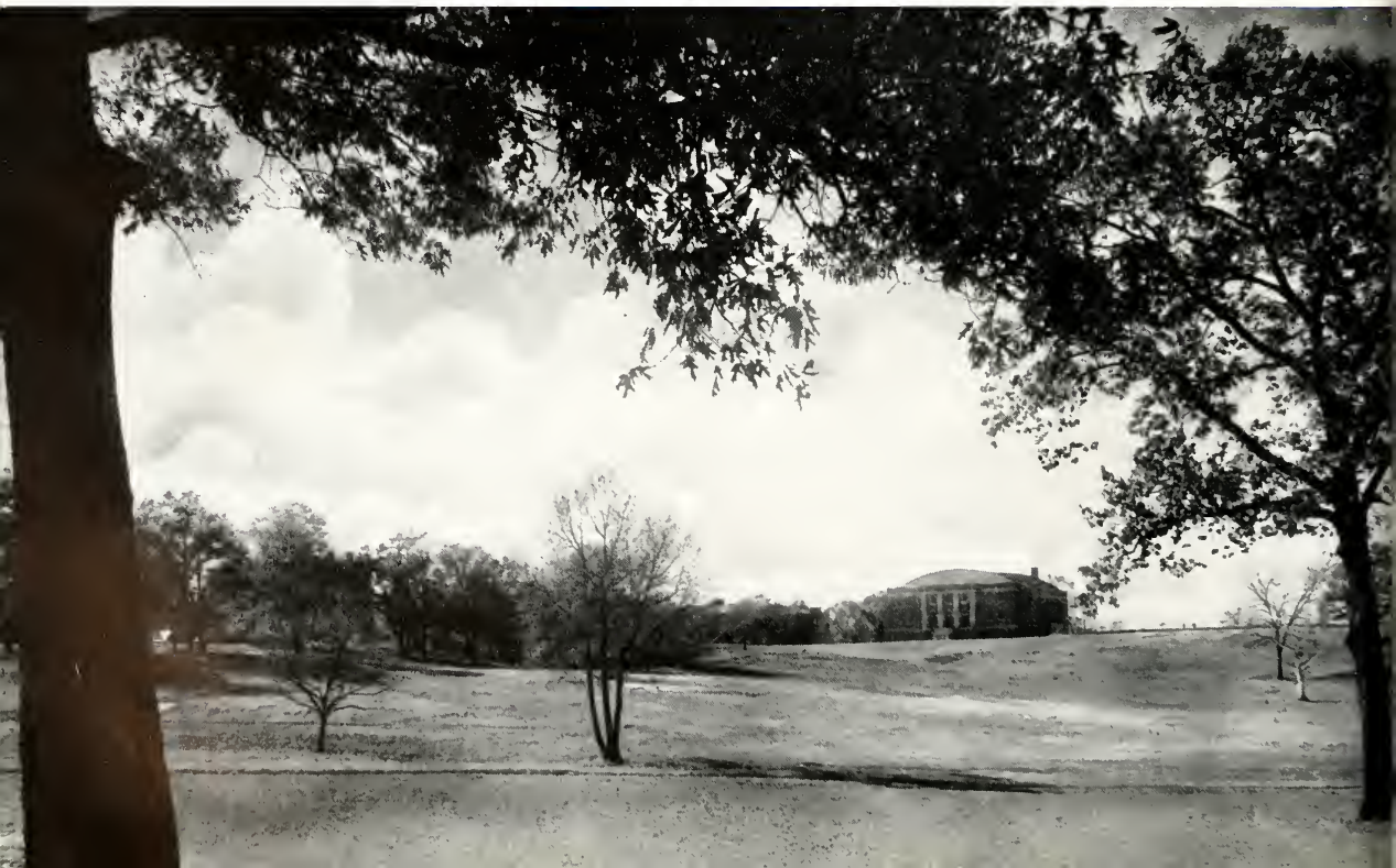
BUIE MEMORIAL GYMNASIUM ●
