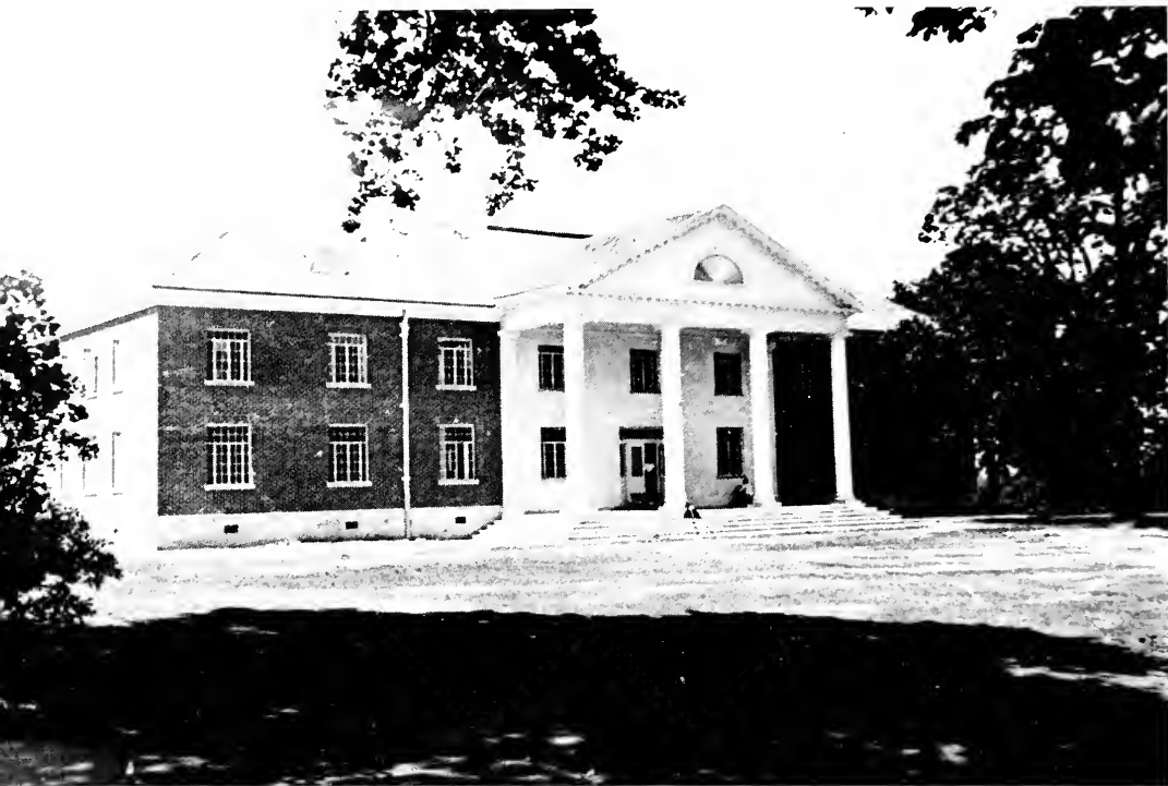
● NEW WOMEN'S DORMITORY
