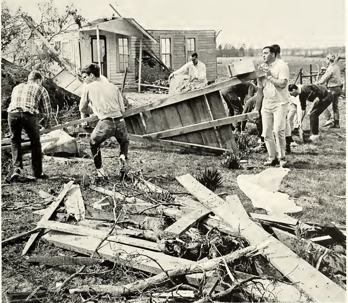
Tornado relief workers clear debris and salvage building material.
