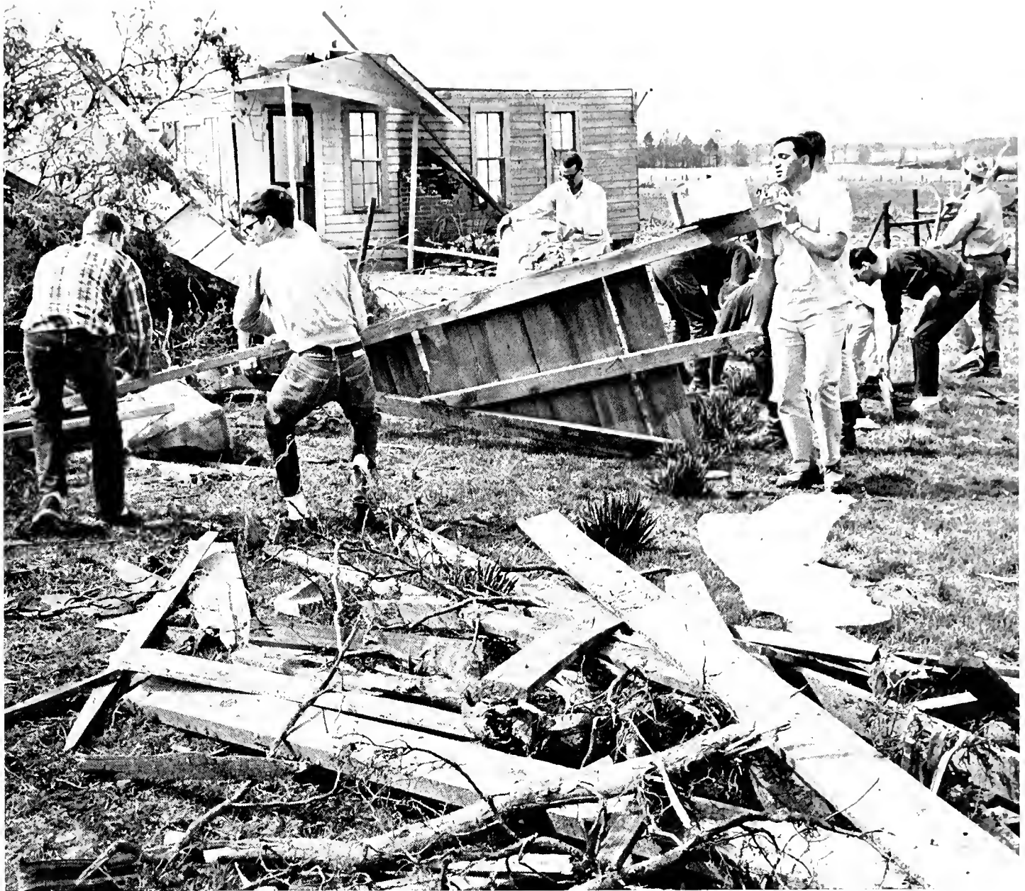
Tarnada relief warkers clear debris and salvage building material.
