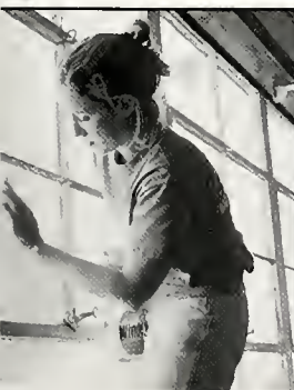
Katie Hardy: House repairs during Delta Delivery
