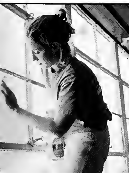
atie Hardy: House repairs during Delta Delivery
