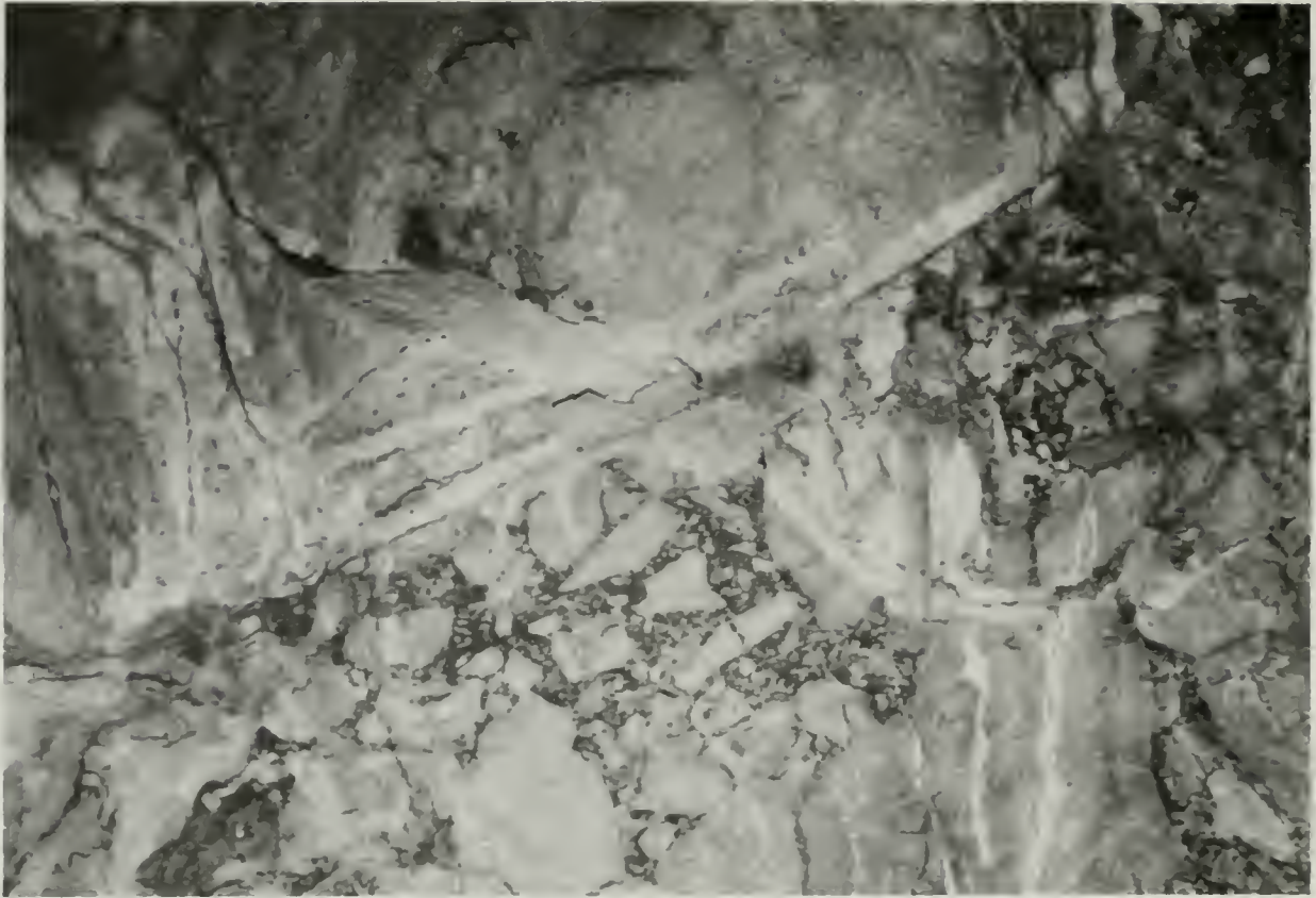
Photo 7. Veined and propylitically altered tuff breccia of the Silver Hill Volcanic Series, as exposed underground in the Bulwer tunnel, about 150 feet west of the contact with the intrusive dacite. Scale is 6 inches long and rests against a pyroclast of argillically altered dacite.
