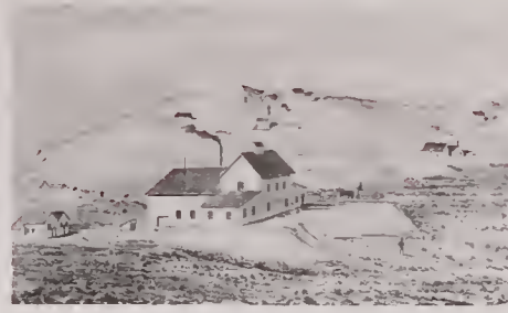
9. Dudley Hoisting Works
