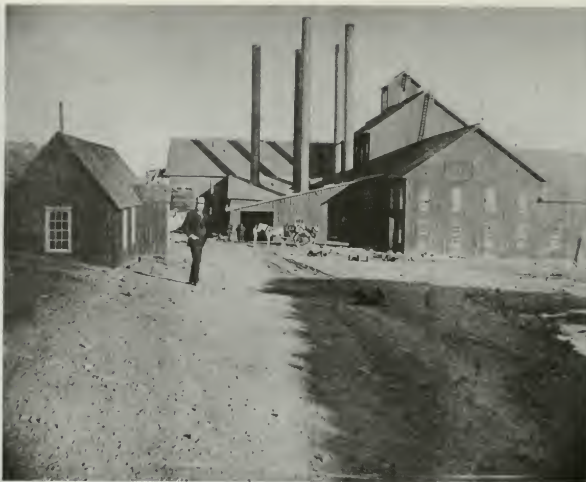
Photo 15. Lent shaft hoist house and office, as it appeared in 1895. Photographer unknown [Frederick, 1960, private communication].
