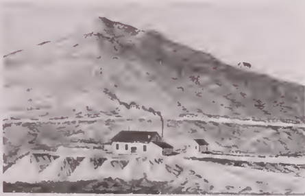
3. The Bodie Tunnel
