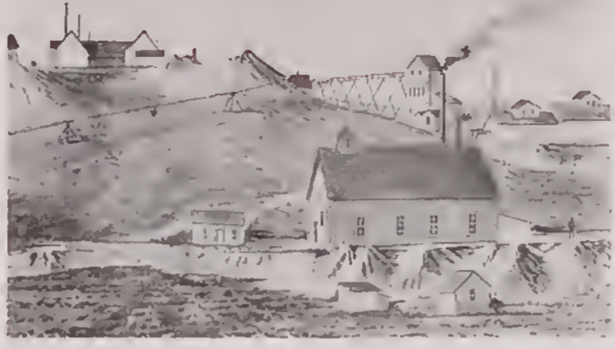
7. South Bulwer Hoisting Works
