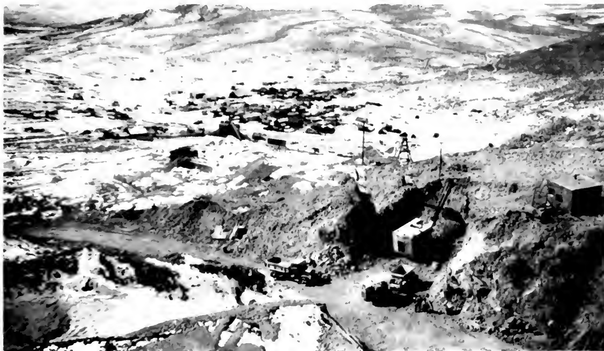
Photo 16. View of Bodie looking southwest from Standard Hill. Excavation in foreground is part of large scale sampling conducted by Yukon-Treadwell Company, Inc. in the Spring of 1931. Photograph by Francis H. Frederick.
