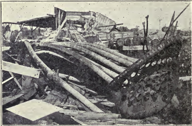
Fig. 7. Close-up view of boiler tubes and head.
