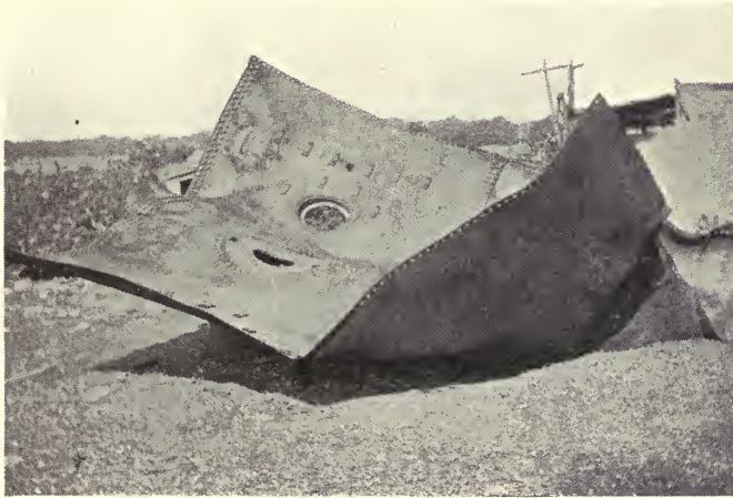
Fig. 2. View of shell plates, showing patch and extent of crack.
