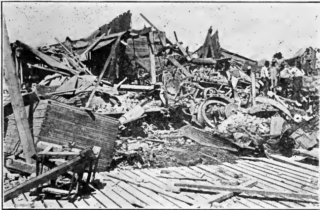
Fig. 6. Result from the explosion of a single-sheet boiler.
