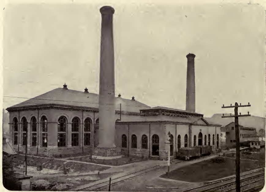
MONTROSE PUMPING STATION, ALLEGHENY, PA.
