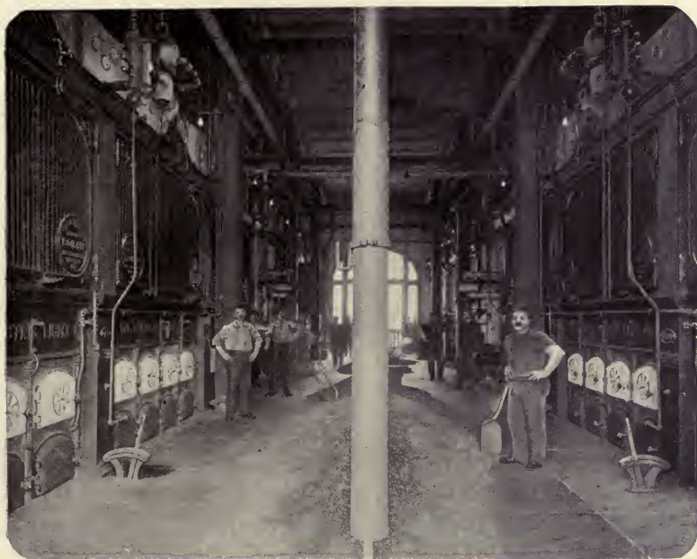
EDISON ELECTRIC LIGHT CO., SANSOM STREET STATION, PHILADELPHIA, PA. Superheating Water-Tube Boilers.
