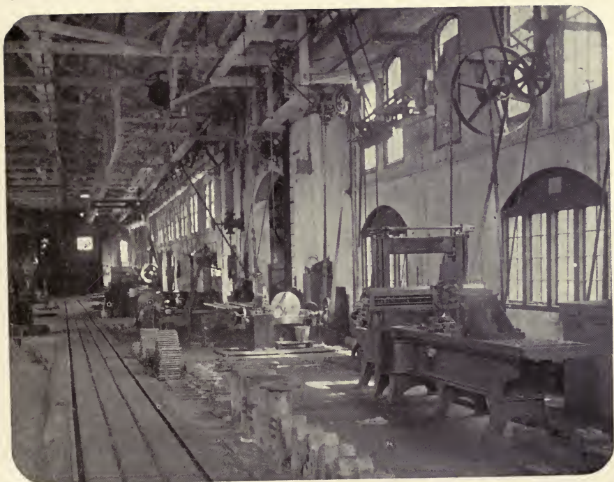
INTERIOR VIEW OF MACHINE SHOP.
