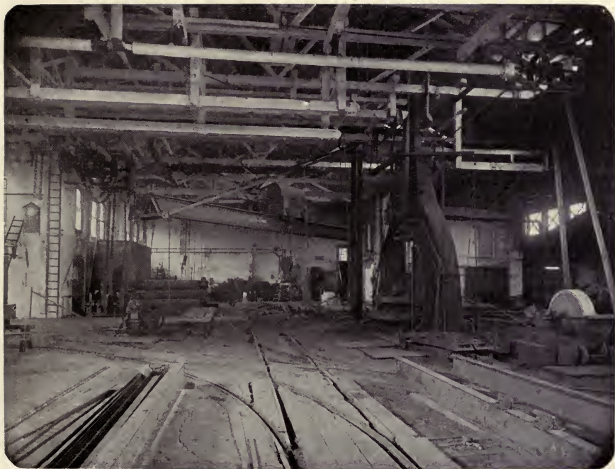
INTERIOR VIEW OF FORGING AND RIVETING SHOP.
