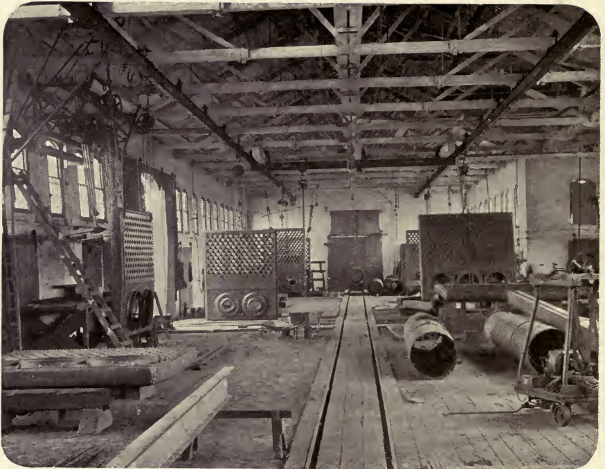
INTERIOR VIEW OF ASSEMBLING SHOP.
