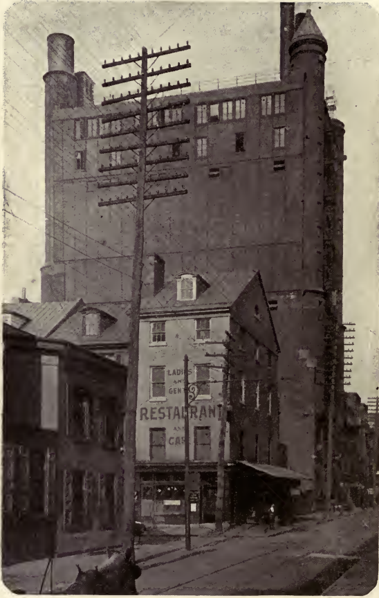
EDISON ELECTRIC LIGHT CO., SANSOM STREET STATION, PHILADELPHIA, PA.
