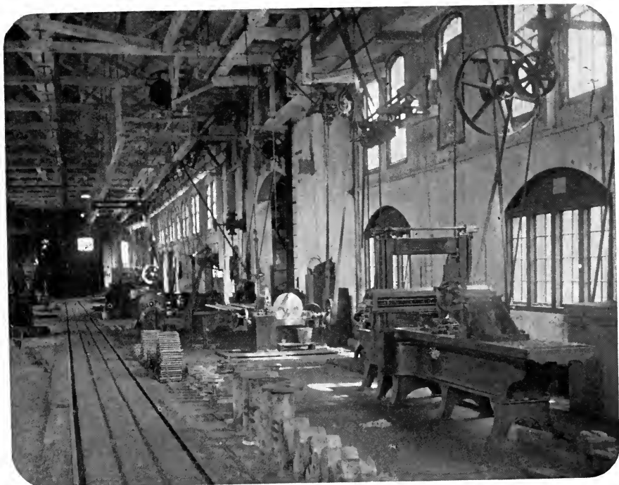
INTERIOR VIEW OF MACHINE SHOP.
