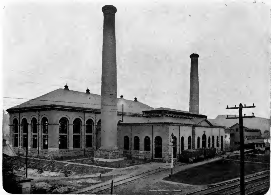
MONTROSE PUMPING STATION, ALLEGHENY, PA.
