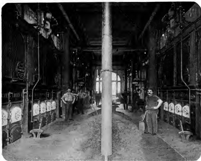
EDISON ELECTRIC LIGHT CO., SANSOM STREET STATION, PHILADELPHIA, PA.
