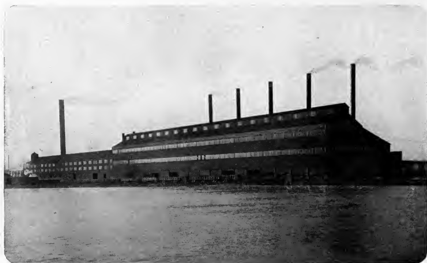
DIAMOND STATE STEEL COMPANY, WILMINGTON, DEL.
