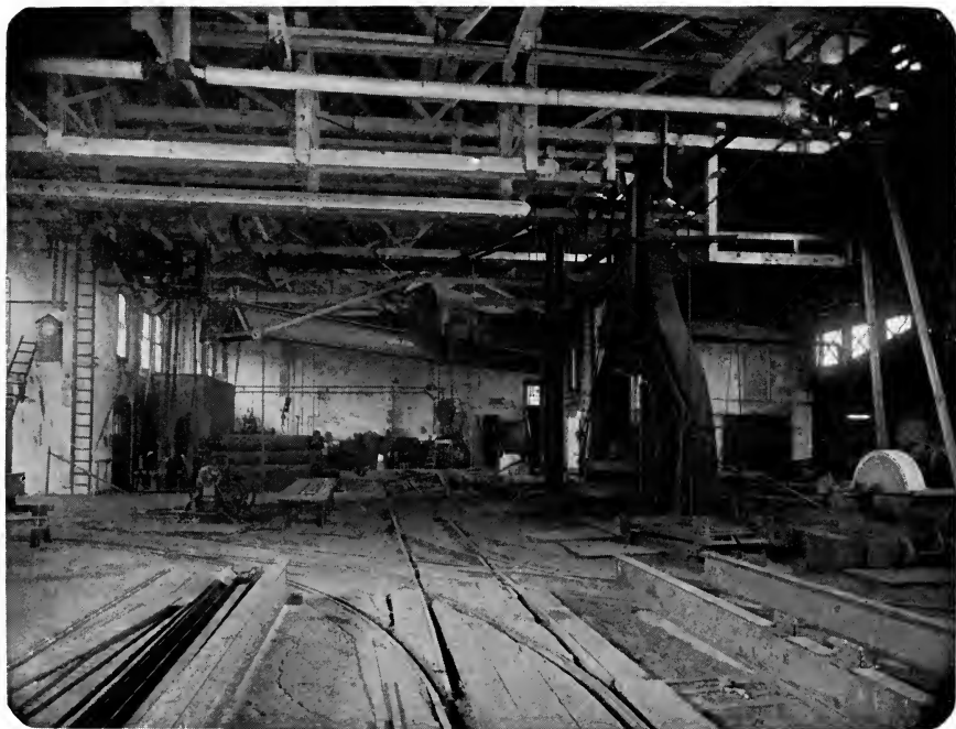
INTERIOR VIEW OF FORGING AND RIVETING SHOP.
