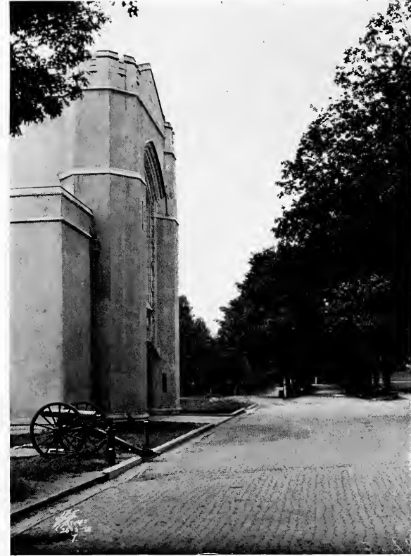
JACKSON HALL AND THE DRIVEWAY
