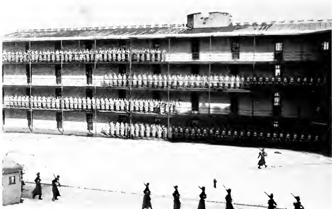
INSPECTION ON STOOPS
