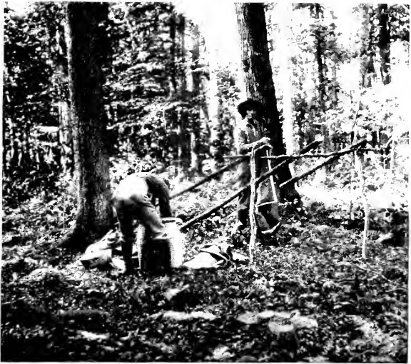
Starting a Lean-to Shelter
